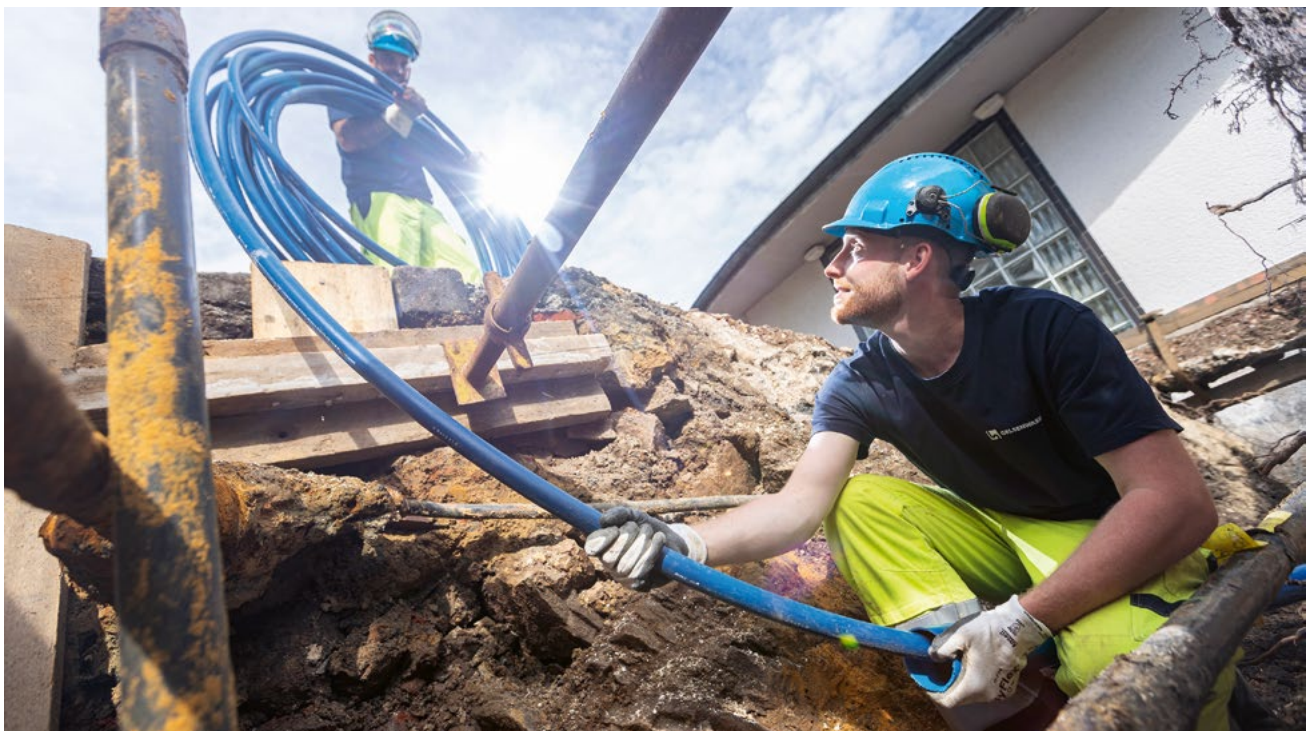
The renewal of the network infrastructure, such as here in Hattingen using the pipe pull-in method, prevents leaks in the pipe network.
